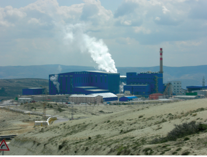
Figure A18 (Stop 18). Beypazarı trona solvay process plant. Detailed information will be given by the staff of the plant.
